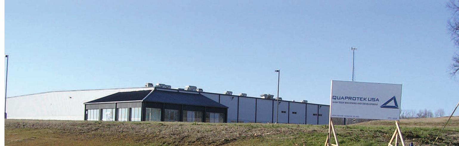
Quaprotek USA has spent the last year getting the former spec building in Ripley ready for production. Not yet finished when this picture was taken is a canopied walkway that extends from the front door over an open moat that was installed to help with drainage.
